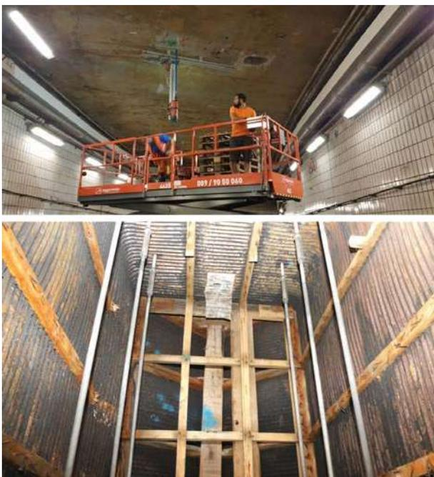
*Figure 8. Installation and installed screw anchors during the preliminary works*
